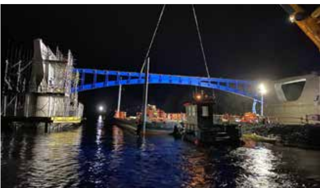
Ballina/Killaloe Shannon Bridge Crossing works in progress
