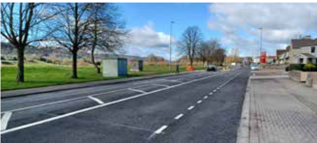
N24 Pavement Improvement Scheme, Clonmel Road Carrick On Suir
