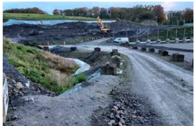
Ballaghveny Landfill - Cell 10B being filled with waste, 9th November 2023
