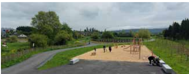
River Ara Walkway Completed
