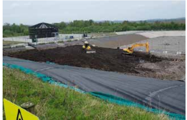
Ballaghveny Landfill - Cell 10B commenced filling, 23rd March 2023
