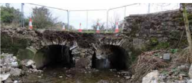
Rehabilitation Works At Gullet Bridge Ballingarry 2023
