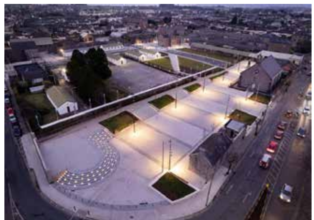
Kickham Barracks Plaza Completed
