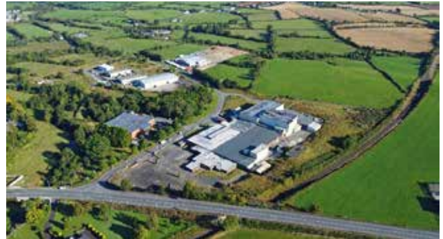
Aerial view of Lisbunny Industrial Estate
