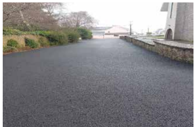
Resurfacing works at Silvermines Church
