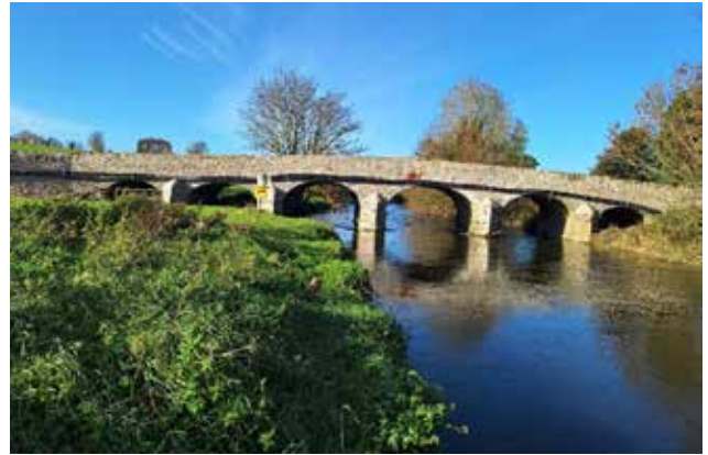
Remedial Works at Annaghbeg Bridge
