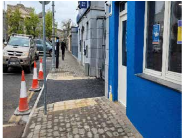
Repair of footpaths at Kickham Street, Nenagh
