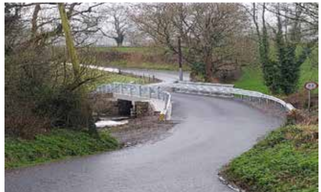
Templederry Bridge - new bridge deck, parapets & safety barriers installed
