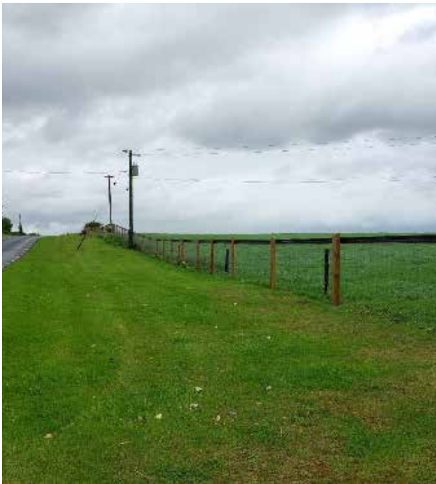
Fencing Retrofit at Tinlough, Carrig
