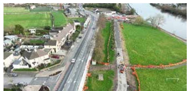
Carrick on Suir Phase 1 Works in Progress
