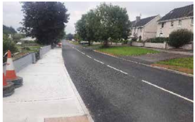
Footpath and resurfacing works at Dromineer
