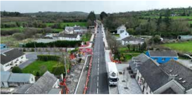
N76 Pavement Improvement Scheme at Grangemockler
