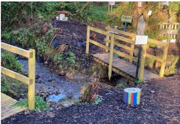
Bridge erected over stream by Shallee Enhancement Group
