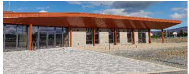
Fethard Town Park Completed
