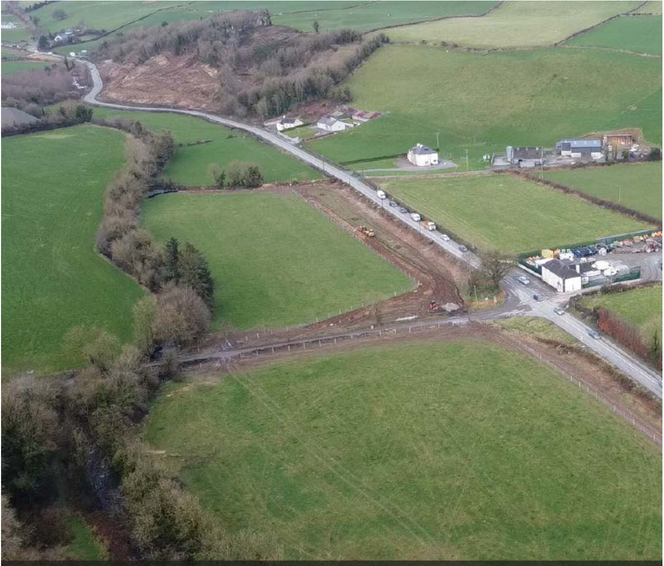
Site Clearance and Fencing in advance of Main Works Contract.
