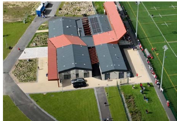
Fethard Town Park Completed
