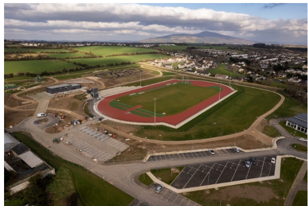
Clonmel Regional Sports Hub Completed
