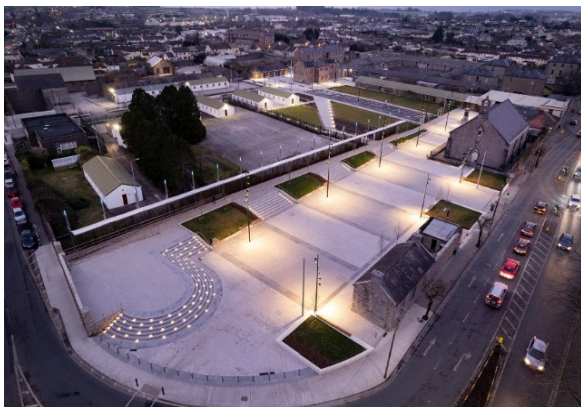
Kickham Barracks Plaza Completed
