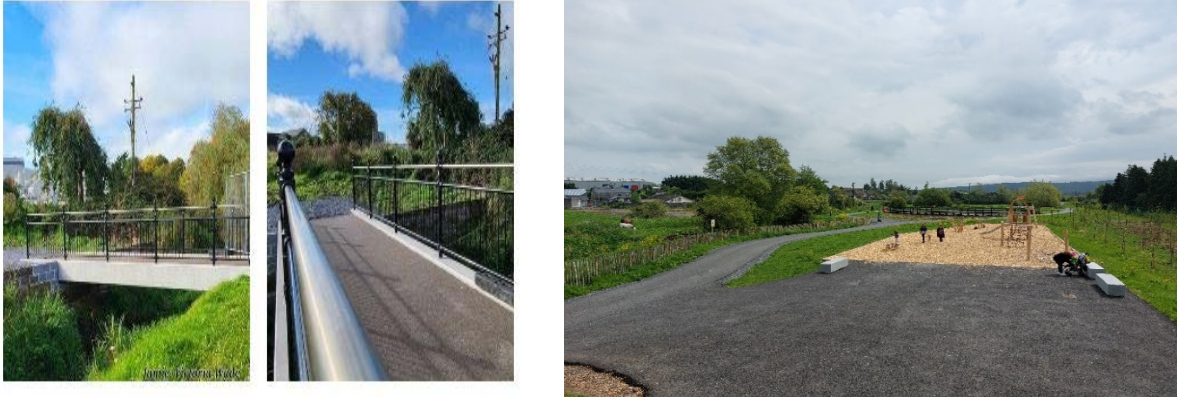
River Ara Walkway Completed
