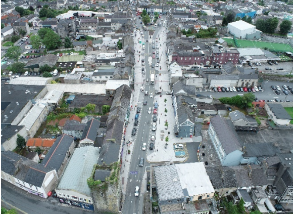
Liberty Square Phase 1 Completed
