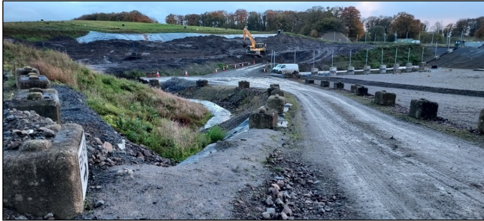
Ballaghveny landfill- Cell 10b being filled with waste, 9th November 2023
