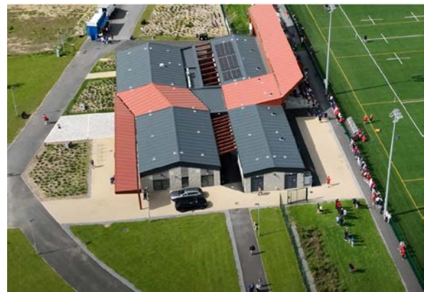
Fethard Town Park Completed
