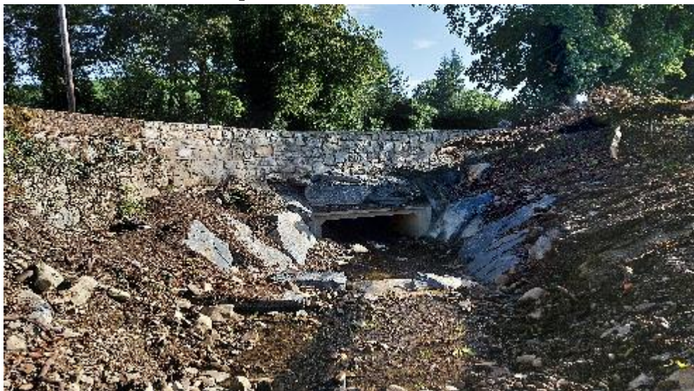
Culvert installation – Curraghnaboola, Borrisoleigh
