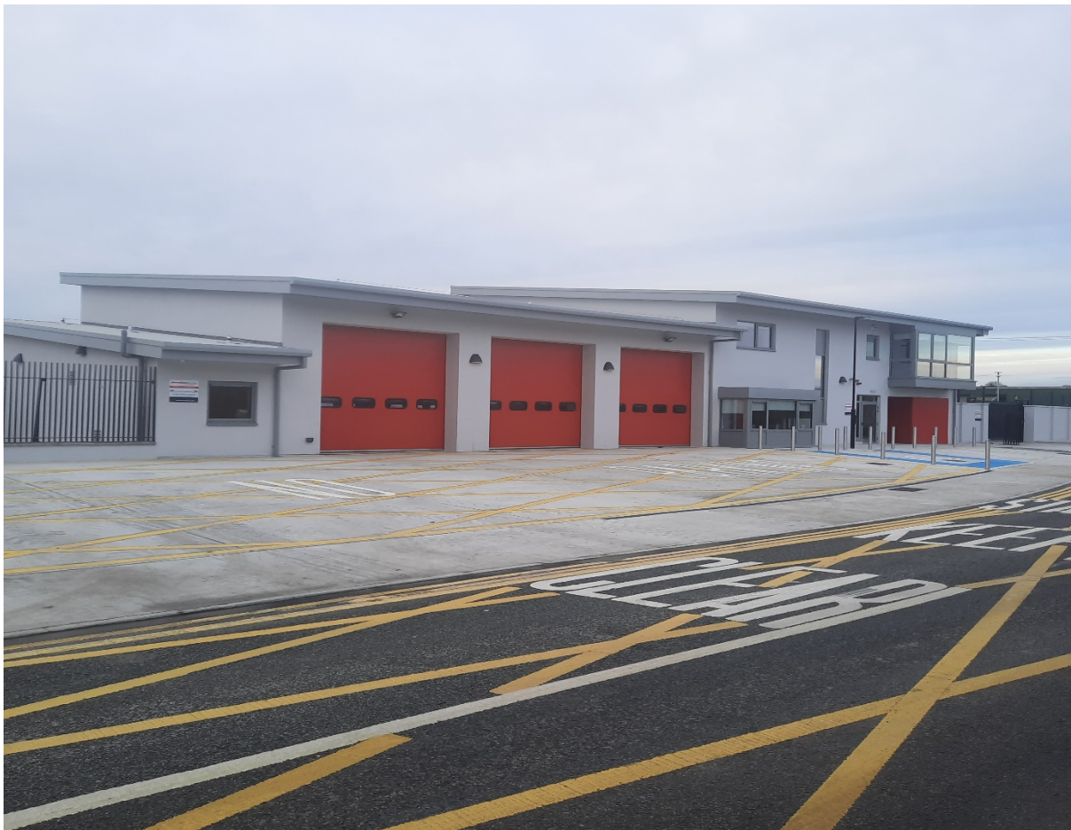
New Cashel Fire Station
