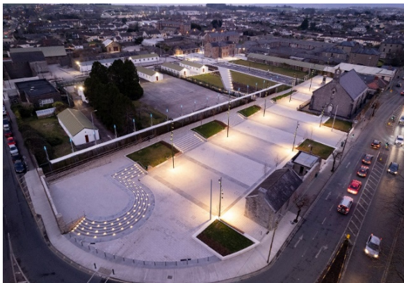
Kickham Barracks Plaza Completed
