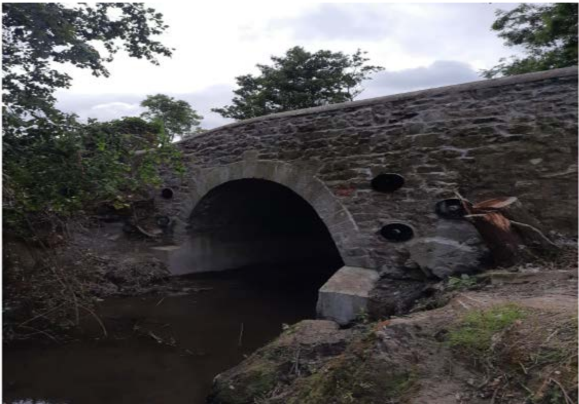
Ballylanigan Bridge – works completed June 2023
