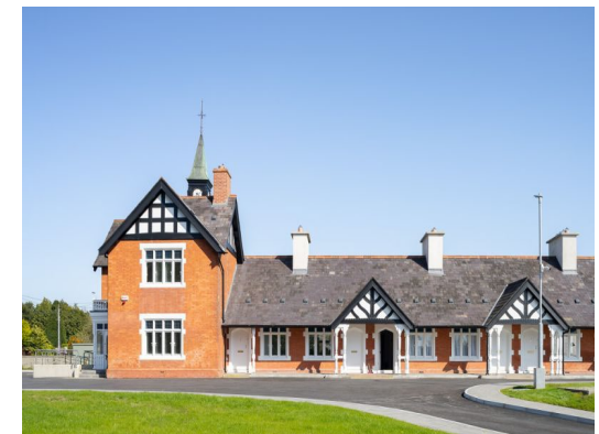
Stanwix Village – Dublin Rd, Thurles Protected Structure
