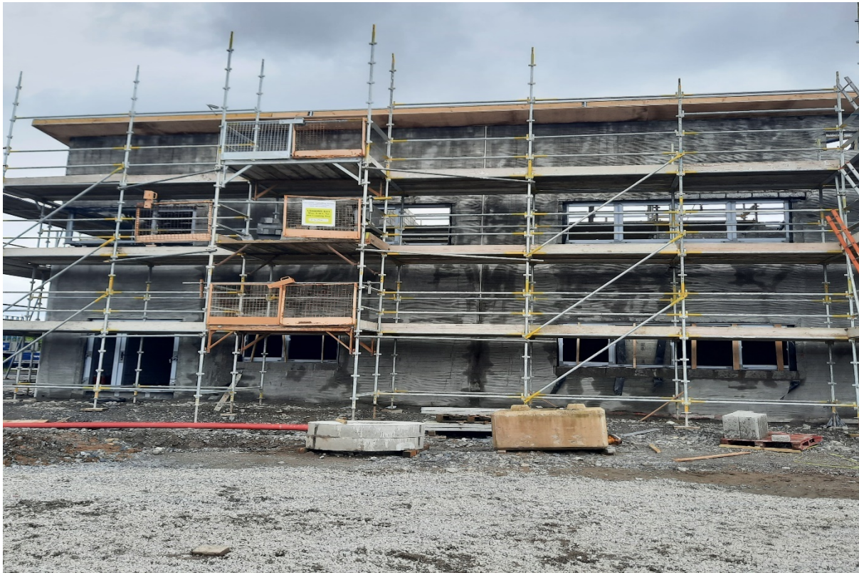
New Cashel Fire Station
