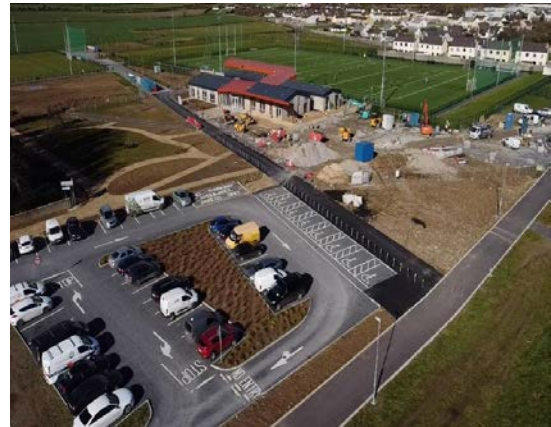
Fethard Town Park Completed
