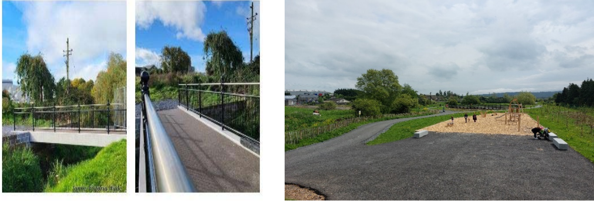
River Ara Walkway Completed
