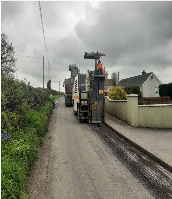
Lisnagrough Road Improvement
