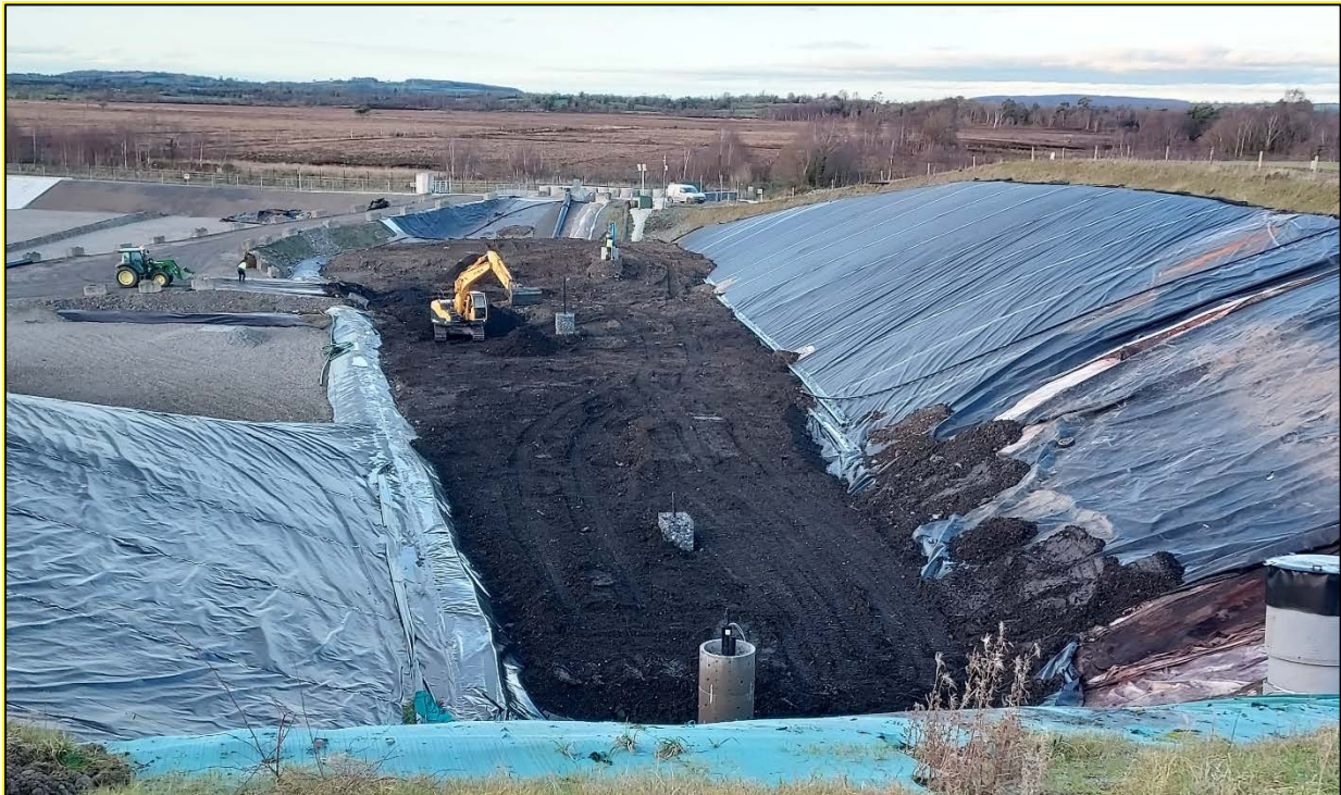
Ballaghveny Landfill - Wedge Cell being filled with waste, 15 th December 2021
