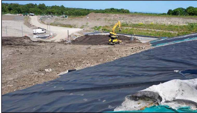
Ballaghveny Landfill – Cell 10b being filled with waste, 30th May 2023
