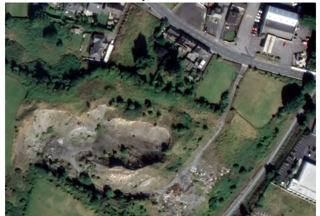
Birr Road Former Quarry, Aerial View
