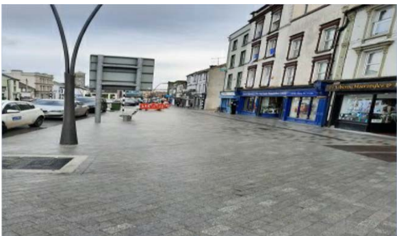
Liberty Square Phase 1 Completed
