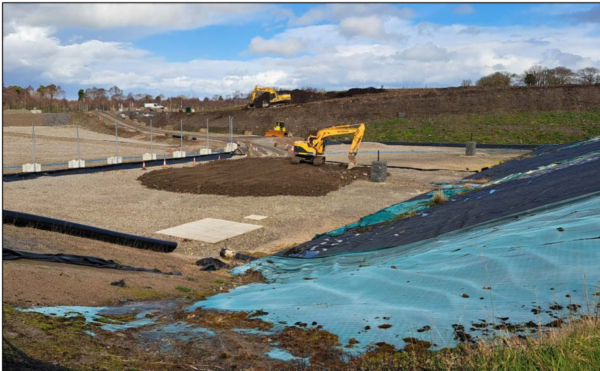
Ballaghveny Landfill – Cell 10b being filled with waste, 23 rd March 2023
