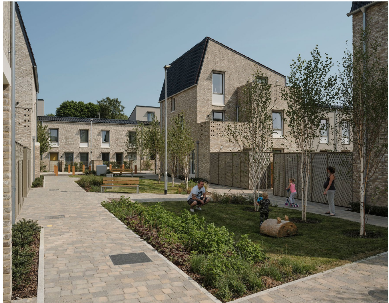
Goldsmith Street, Norwich - High density, sustainable housing with a focus on pedestrian use
