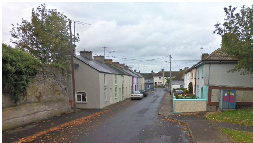
Ikerrin Road streetscape and buildings looking north
