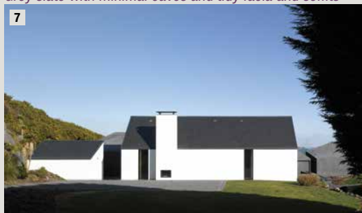
Grey slate with minimal eaves and tidy fascia and soffits
