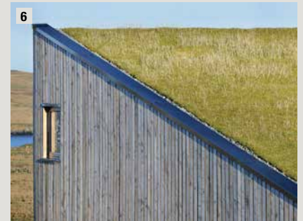
Green roof coverings
