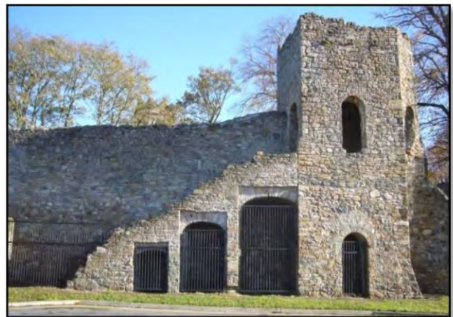
Figure 7.5 Exterior of Clonmel Town Wall at St Mary's
