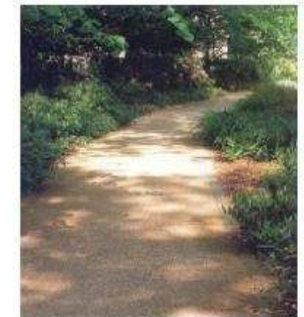
Self binding gravel informal paths of open spaces
