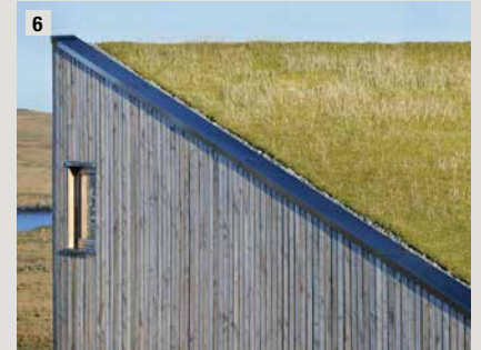
Green roof coverings
