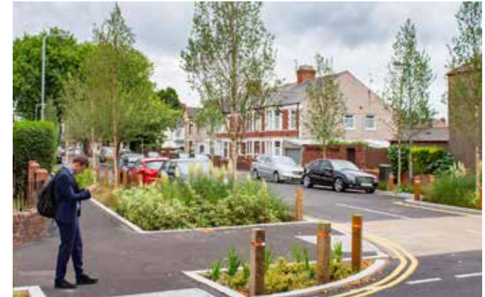
Large hardscape areas and roads means that drainage infrastructure is often at or above capacity. Heavy downpours result in the system being overwhelmed resulting in flooding and associated pollution and damage. Greener Grangetown in Cardiff is a very interesting example of the successful retro installation of sustainable urban drainage system features into an existing urban streetscape. Retrofitting street trees, and, within an existing residential neighbourhood road. Source: GreenBlue Urban
