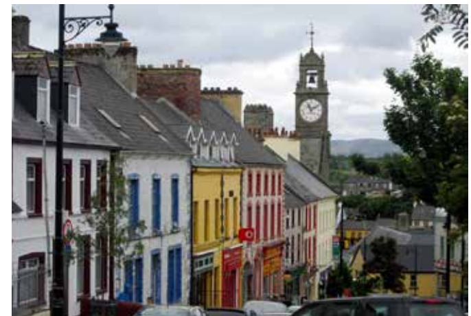
Ballyshannon Design Guide: The guide highlights areas of distinctive character and other qualities valued in the town; and assists in the task of maintaining, repairing and restoring existing buildings. Source: Ballyshannon Design Guide
