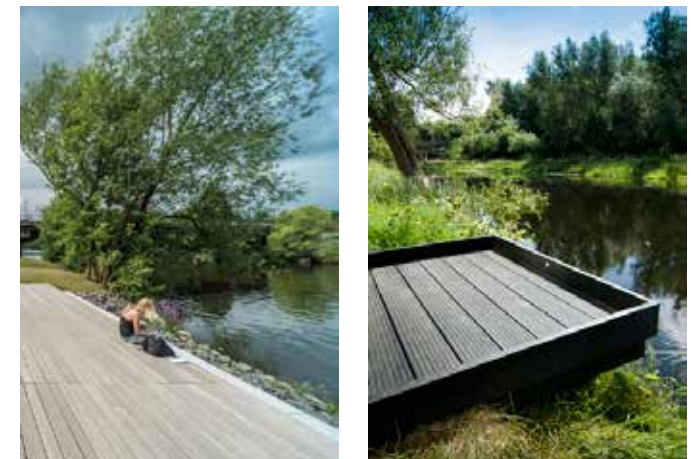
Riverside timber platforms, to provide connectivity and interaction with the river for activities such as fishing. Source: Landezine.
