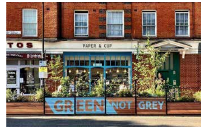
The parklet was built in 2017 to form part of the Shoreditch Low Emission Neighbourhood scheme. The space provides raised wooden planters with lush perennial planting and small multistem birches, as well as climbers which take advantage of the metal railings. The parklet is still in place and functioning today, primarily being used as a spill-out space for the adjacent cafes. Source: Meristem Design
