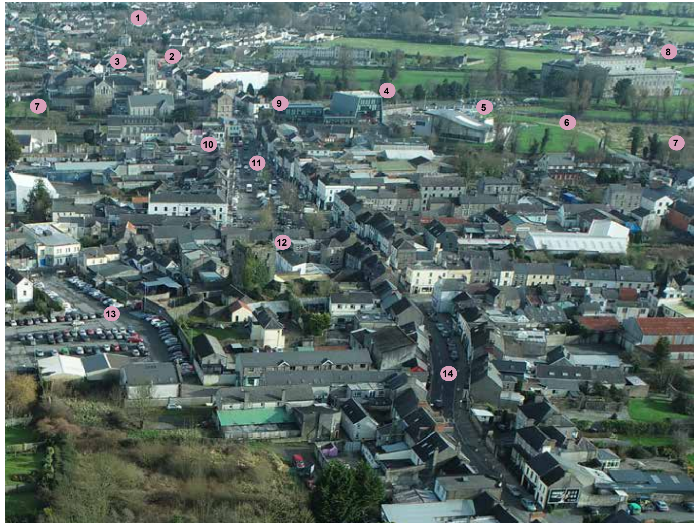
Aerial view of Thurles Town Centre. Source: Tipperary County Council
