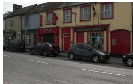
19 th Century Shop Facade
