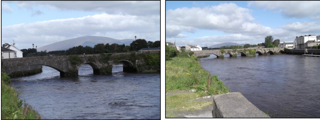
Figure 9: Views of the Old Bridge from the banks of the River Suir
