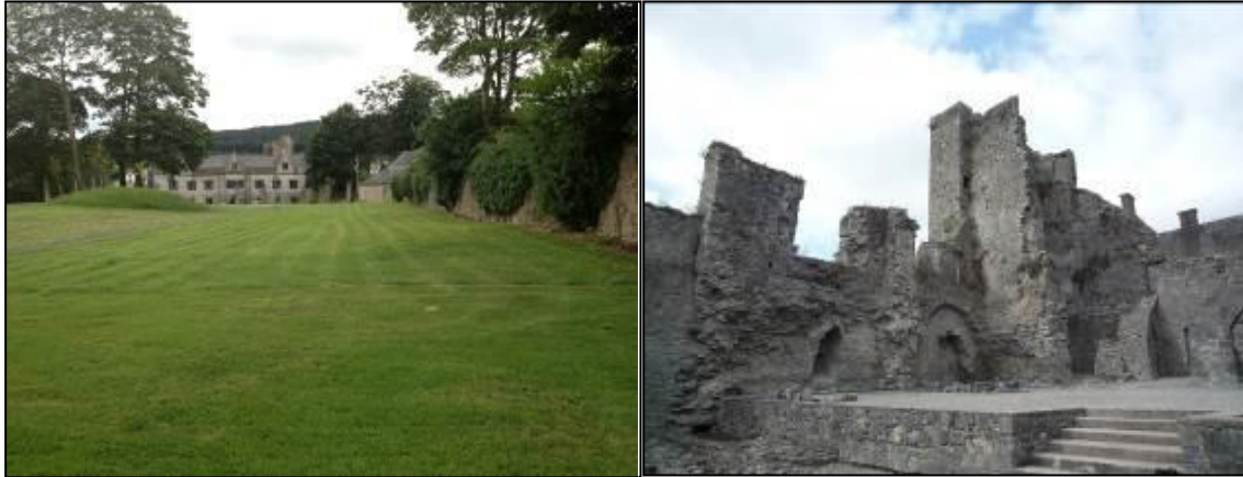
Figure 3: Images of both the exterior and interior of Ormond Castle
