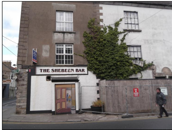
Figure 11: Shebeen Bar and adjoining derelict structure
