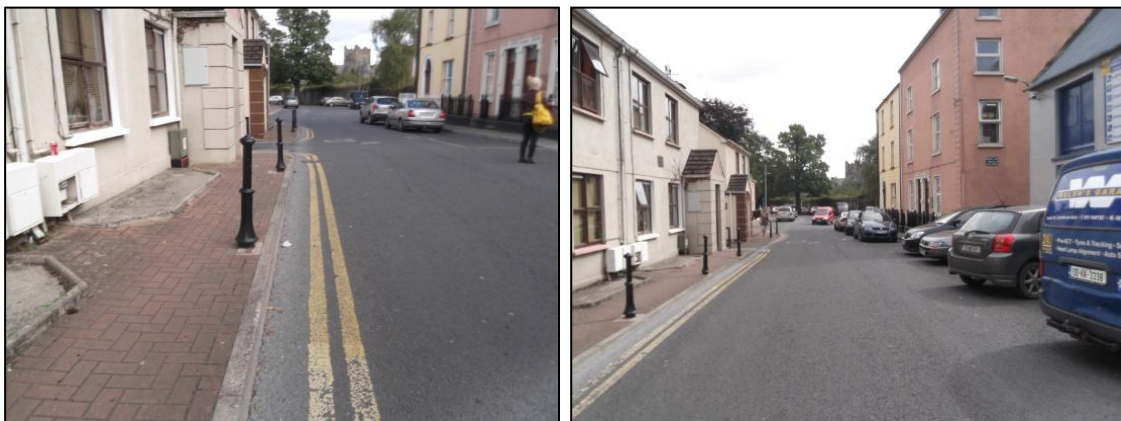
Figure 15: Narrow footpaths and unauthorized parking on Castle Street
