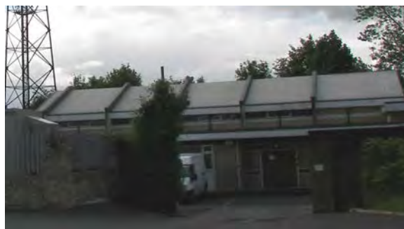
4. Eircom entrance from the central square
