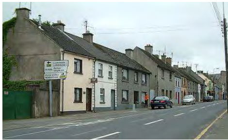
Access points to site from Thomas MacDonagh Street
