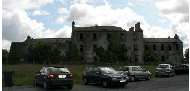
Main Barracks Building with central square and green
