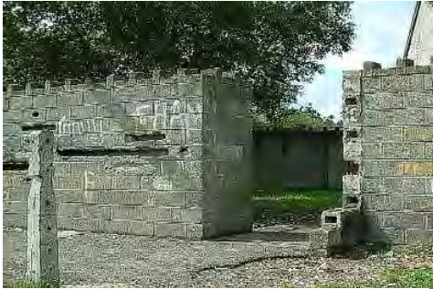
Pedestrian access via Cormack Drive
