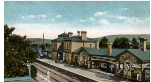
Figure 2.6 Clonmel Railway Station
