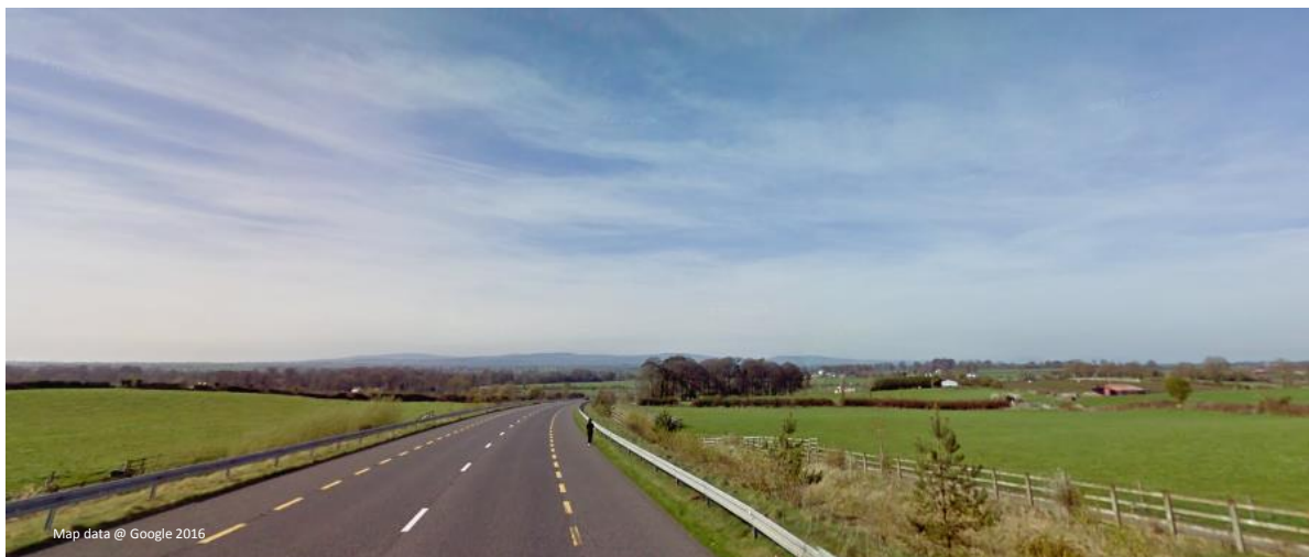
1. View from N74 in Deerpark south west of Cashel [52°30'31.7"N+7°54'31.3"W]
