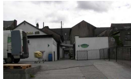
Access to Freshfields and Main Street
