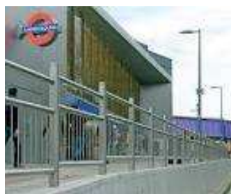
Example of traditional railings
