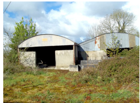
FIGURE 6: AVOID BUILDING CLOSE TO FARMYARDS
