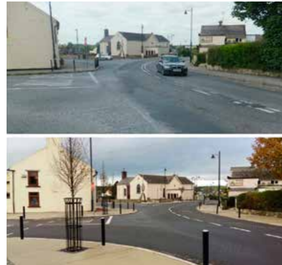
Before and After Works at Ballyclerihan Village.
