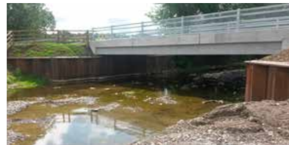
New 14metre single span RC Bridge at Lismalin.
