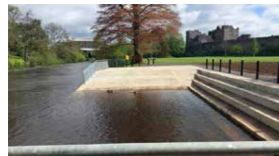
Canoe Steps and Slipway Inch field Cahir
