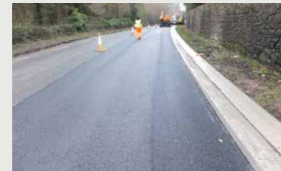
Pavement Re-construction Works at Kilshane during 2015
