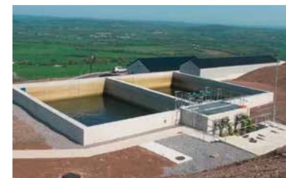
The new Fethard Water Treatment Plant under construction.
