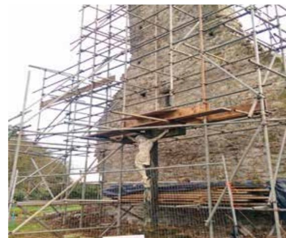
Figure 3 Restoration works on Medieval Church at Modeshil Burial Grounds:
