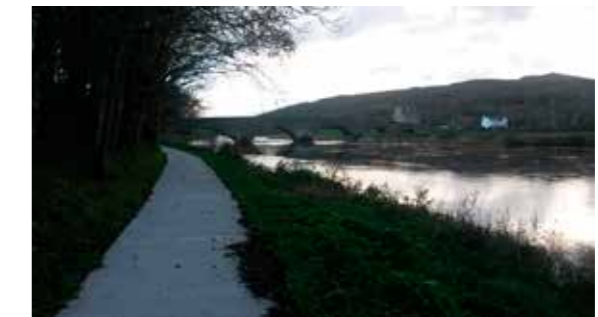
(Photo of completed Greenway footpath/cycle track at Ferryhouse Clonmel – Sir Thomas's Bridge in background)
