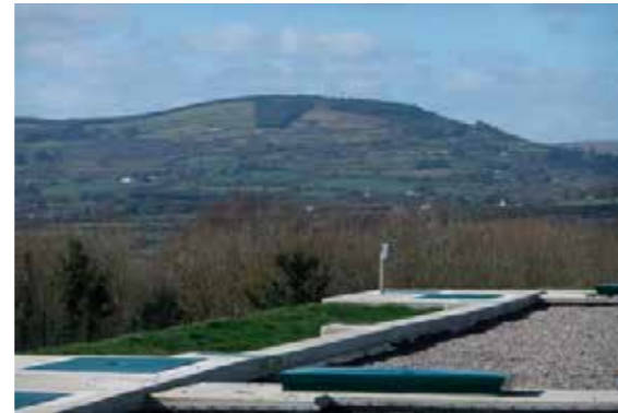
View the old from the new - Knockalough from Garrynamona Reservoir located at Garrynamona, Ballycahill, Thurles, Co. Tipperary
