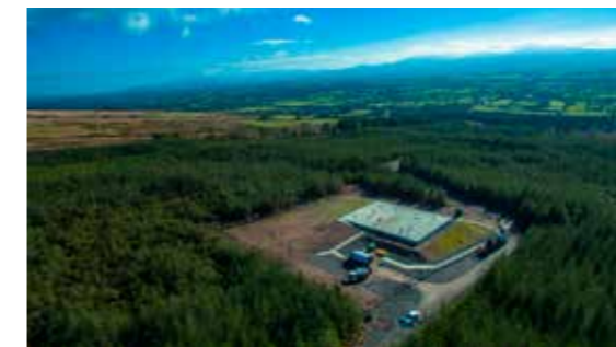
The new Burncourt Water Treatment Plant under construction
