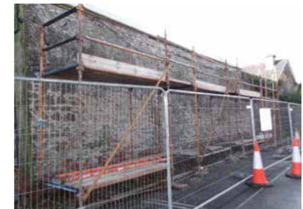
Works in progress in Cashel
