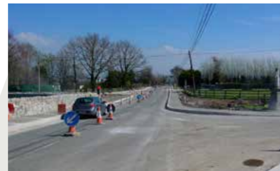
Traffic Calming Works at Thomastown during 2015
