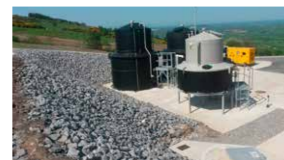
The new Fethard Water Treatment Plant under construction.
