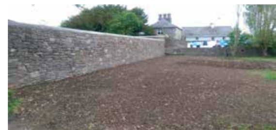
Figure 1.Repaired boundary wall at Emly Burial Ground
