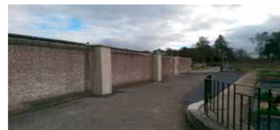
Figure 2 Repaired boundary wall at Cahir Burial Ground
