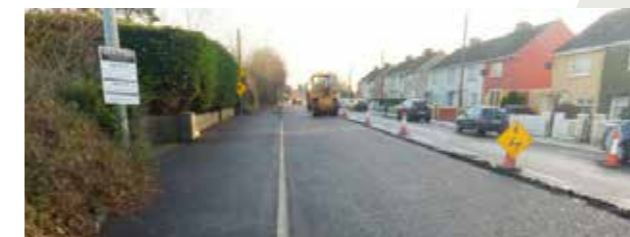
Works at Scart, Roscrea
