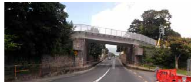
The rail bridge on the N24 Pill Road, Carrick-on-Suir following completion of the works
