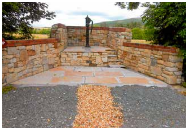
Refurbishment of Village Pump in
