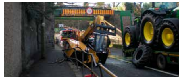
Example of damage caused as a result of a bridge strike at Pill Road, Carrick-on-Suir
