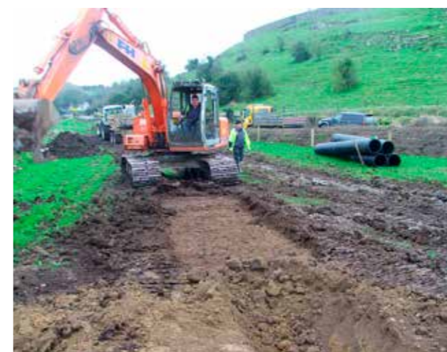
Laying of Lighting ducts
