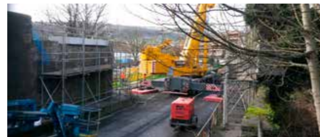
Construction Works on N24 Pill Road, Carrick-on-Suir Rail Bridge February 2017
