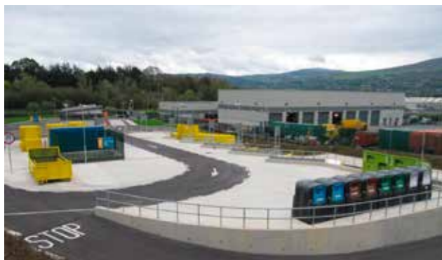
The Clonmel Recycling Centre was shortlisted for the PAKMAN Bring Centre of the year award in association with REPAK.
