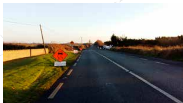
Photo after construction on the N62 Pavement Overlay works at Kilkillahara
