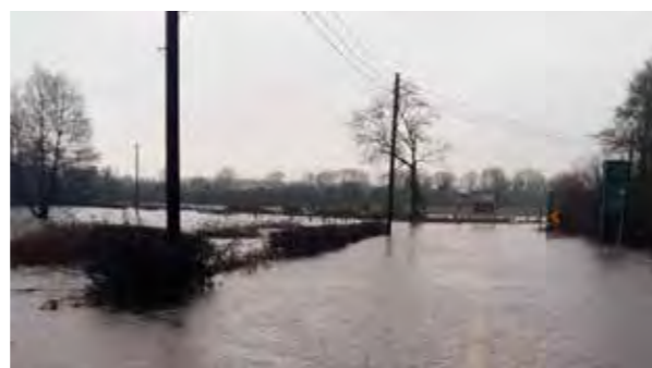
N65 Carrigahorig: Section of flooded road. There is currently a scheme in design to alleviate this.
