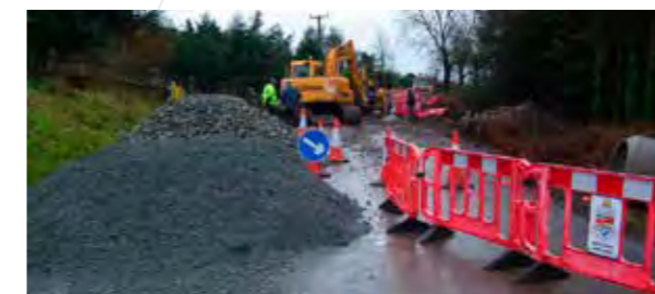
Work being undertaken to alleviate the road slippage at Curraghmarky.
