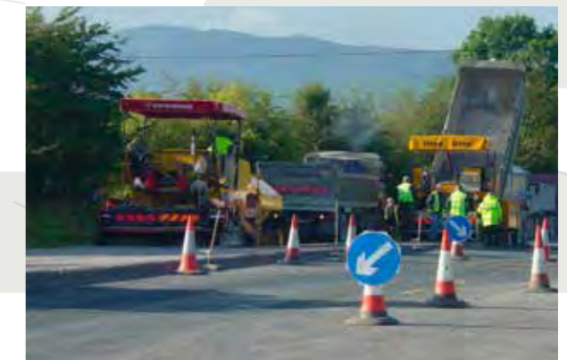
Road Strengthening during 2016
