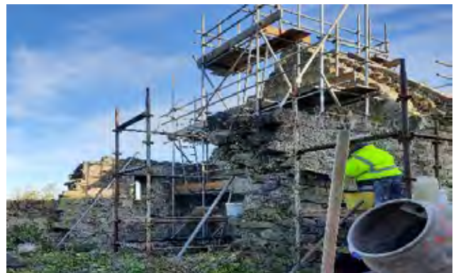
Works in progress Pallas/Dorrha Church
