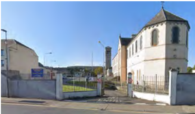
BEFORE - Single Exit At St. Nicholas Carn Park, Greenside, Carrick-on-Suir
