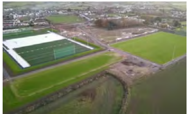
Phase 1 Of Fethard Town Park (Looking South)
