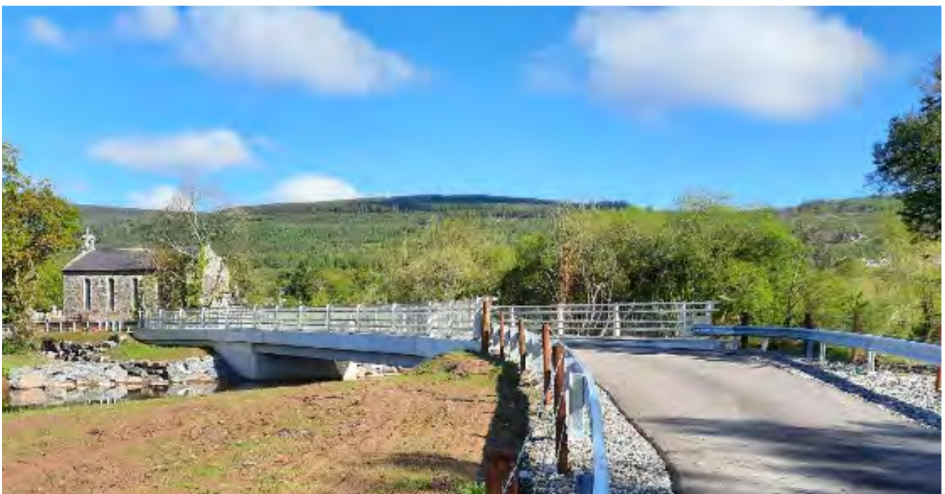
The completed bridge with Clonbeg Church in the background
