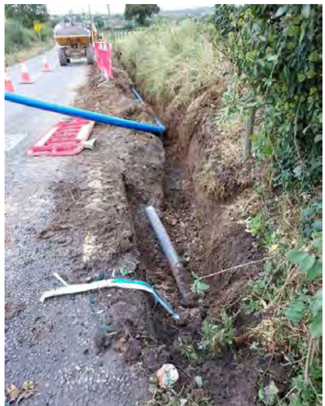
Kilfeacle to Thomastown watermain rehabilitation 02 September 2021
