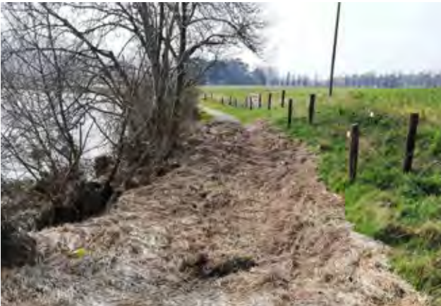
(Clearing of debris on the Blueway after flooding subsides.)
