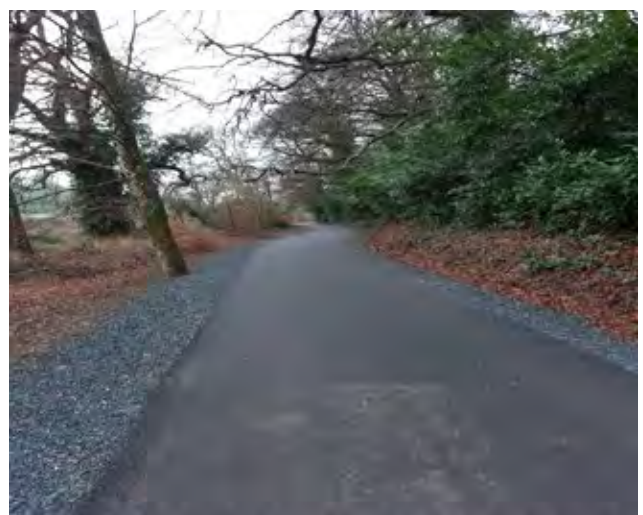
The finished Swiss Walkway in Cahir
