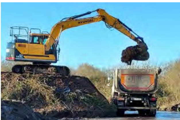
Rathcabbin - stabilised waste being loaded for transport to Ballaghveny landfill
