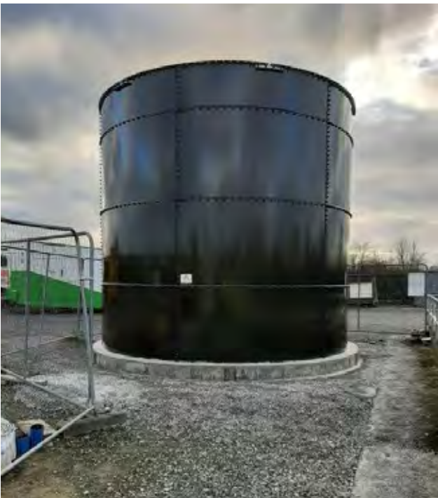
Borrisokane Wastewater Treatment Plant Upgrade Decemeber 2021
