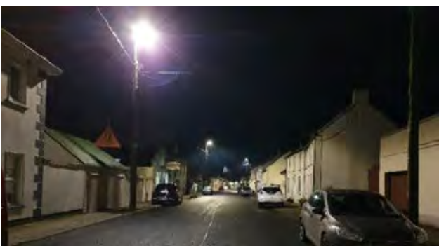
Drangan lighting after upgrade
