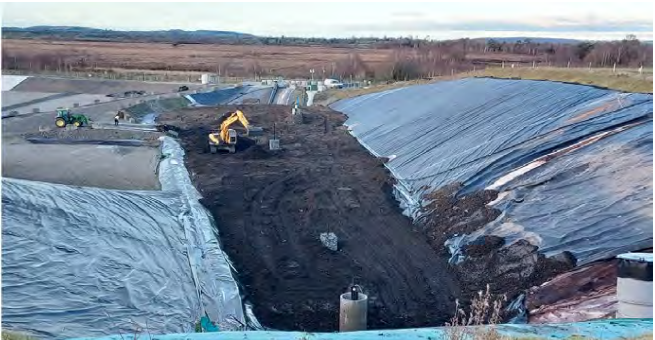
Ballaghveny Landfill – Filling of the Wedge Cell with waste
