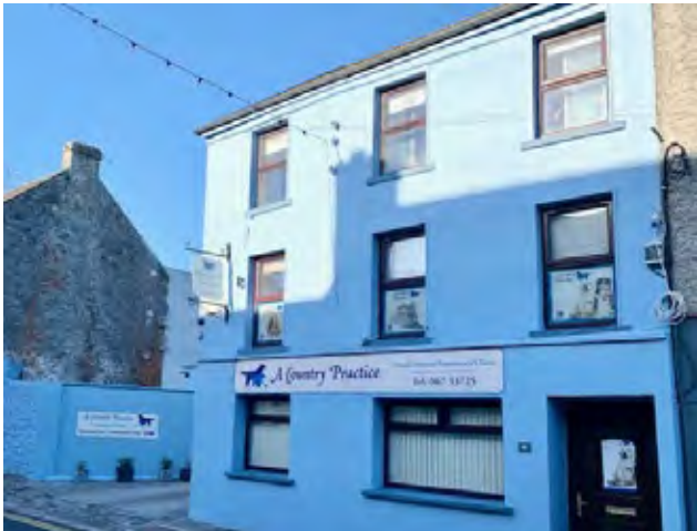
Streetscape scheme work completed
