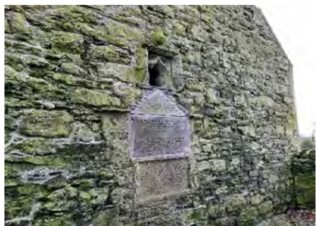
Reinstated repaired plaque
