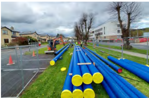
Carrick-on-Suir watermain rehabilitation April 2021
