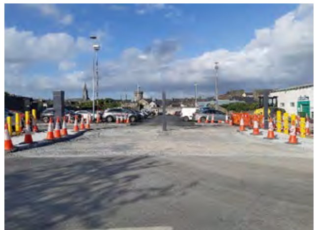
Entrance to John's Lane car park during works
