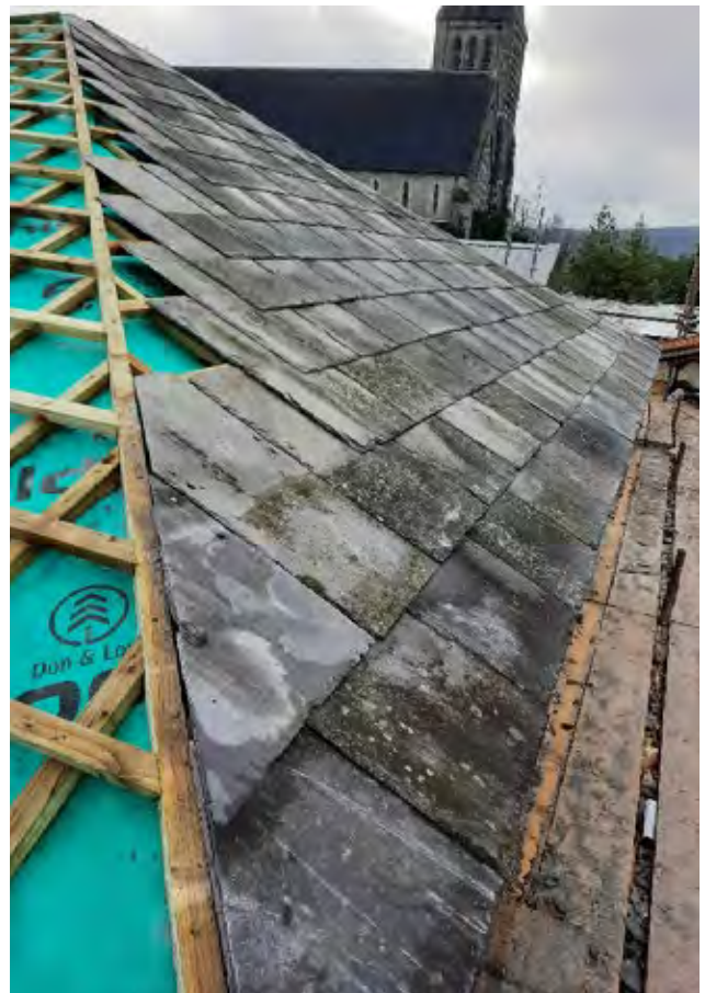
Works progressing at the old Tipperary Town Courthouse
