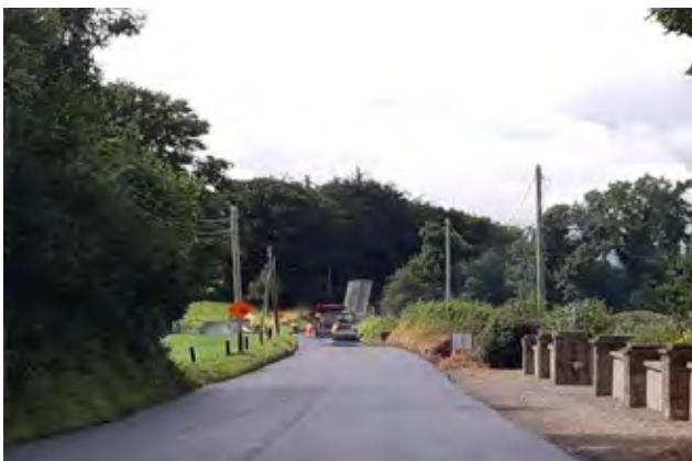
Wetmix works in Grenanstown, Toomevara
