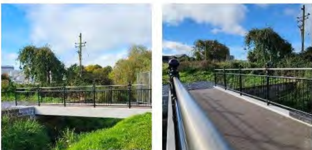
The New River Ara Pedestrian Bridge
