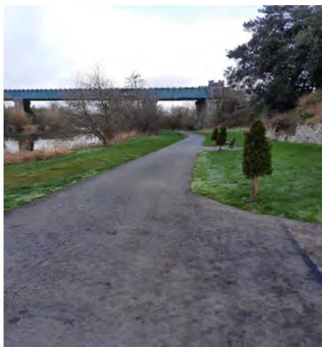
The completed Viaduct Walkway in Cahir
