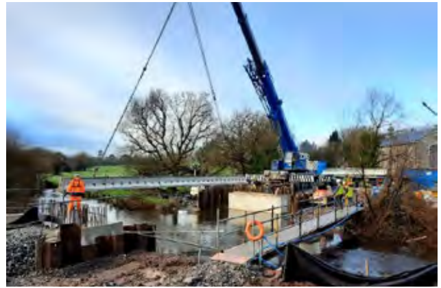
Installation of the Precast Bridge Beams
