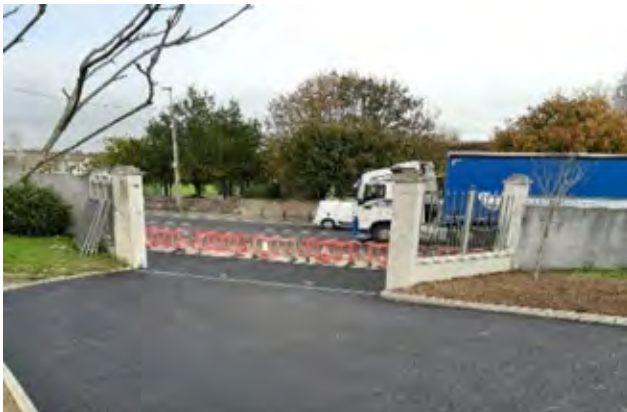
AFTER - New Widened Entrance/Exit At St. Nicholas Car Park
