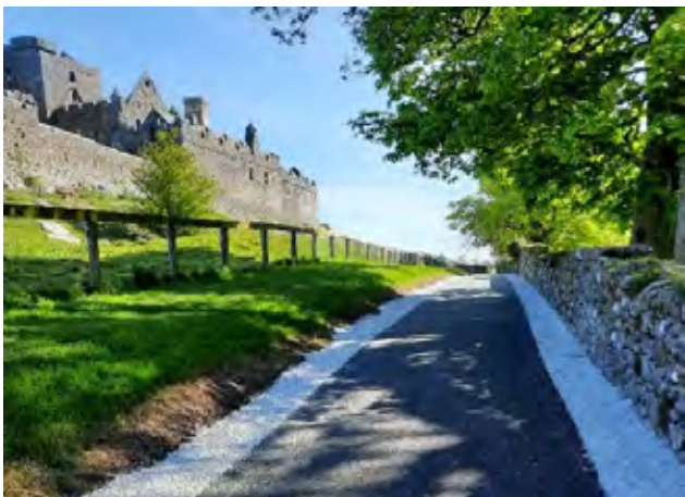
The completed walkway at Bothar na Marbh Cashel
