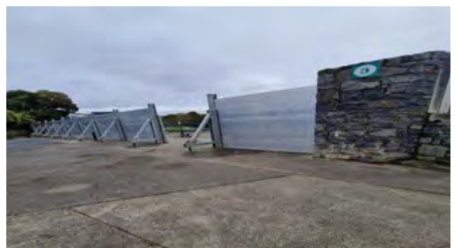
(Flood barriers are installed during flooding season and is a specialized operation. The barriers are left in place until the threat of flooding subsides.)
