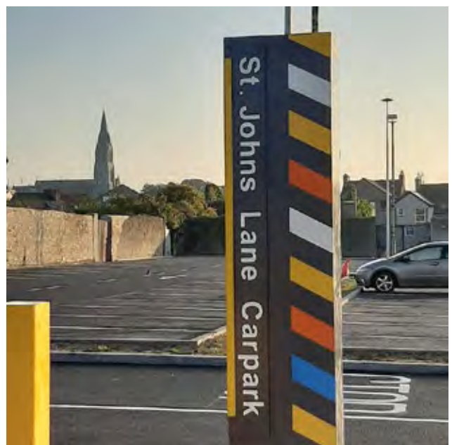
Entrance feature at John's Lane car park after works
