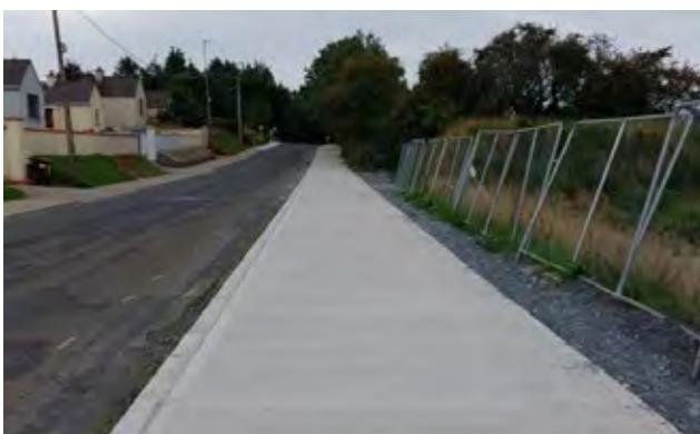
Footpath improvement works at Newport
