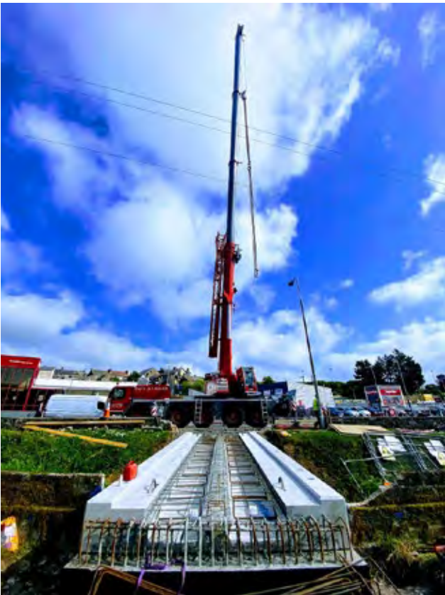
Installation of the Precast Bridge Beams
