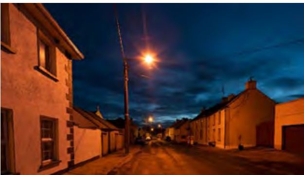
Drangan lighting before upgrade
