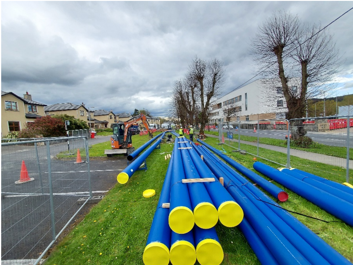
Watermain Rehabilitation at Carrick-on-Suir
