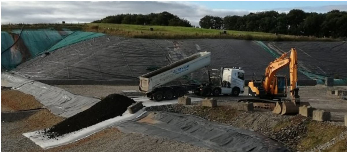
First truck offloading at Ballaghveny
