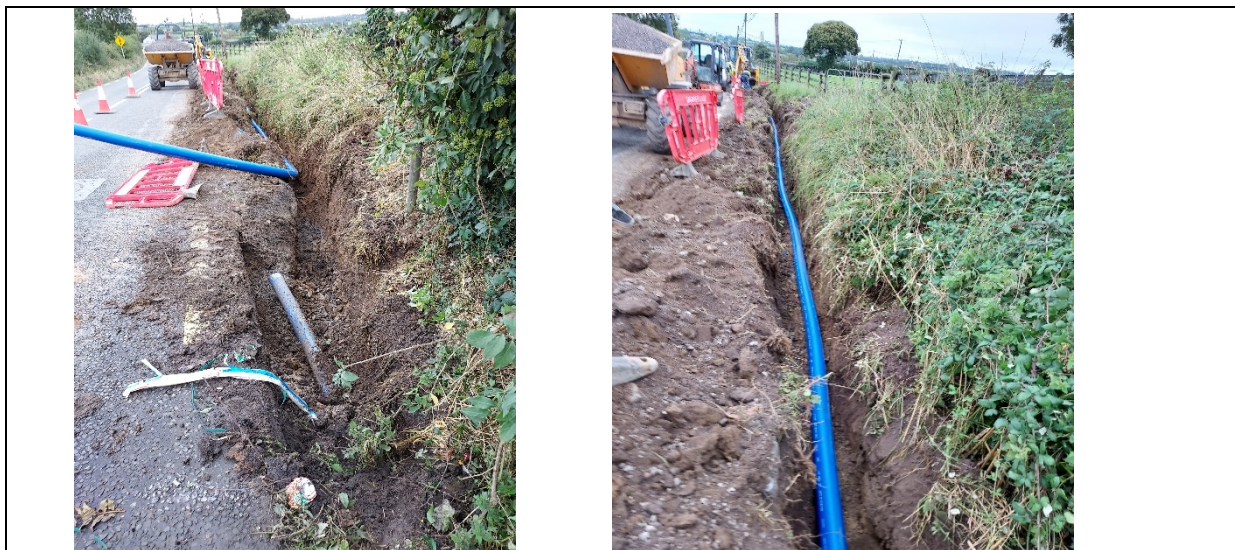
Works at Kilfeakle Thomastown
