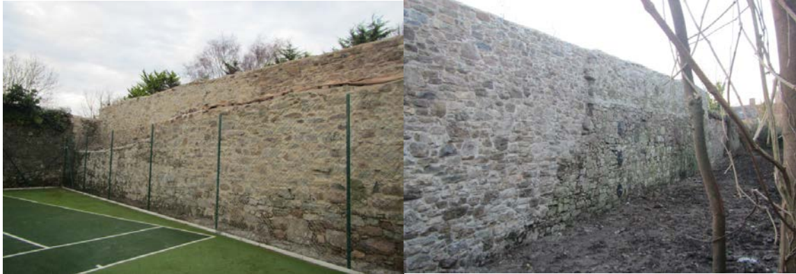
Figure 1: Works complete at Carrick on Suir
