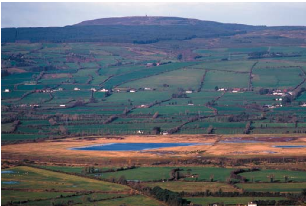
Tailings Management Facility at Gortmore
