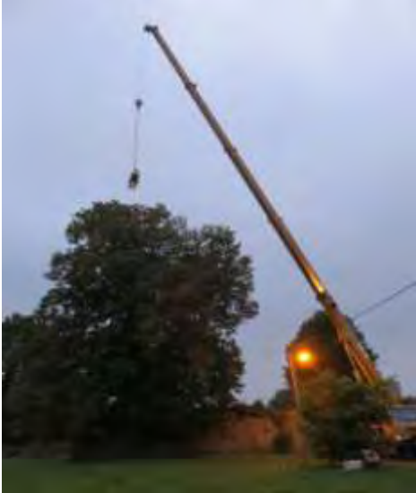
Fig. 3) An early start was made in removing the larger tree.
