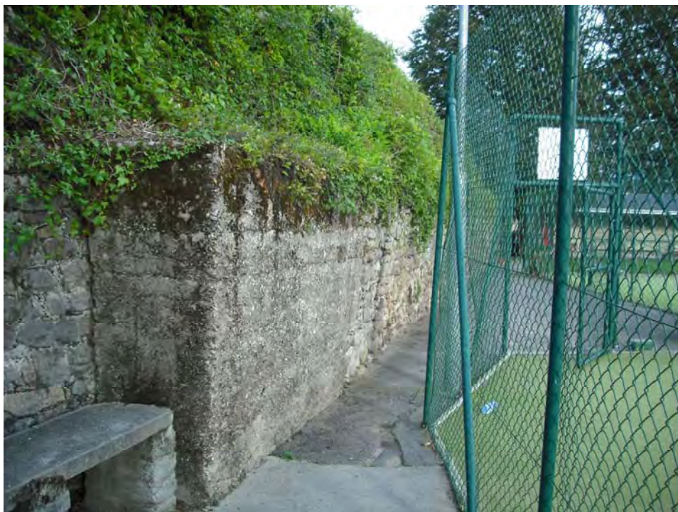
Picture 10 Tennis Court Side Open Concrete Repair Wall A
