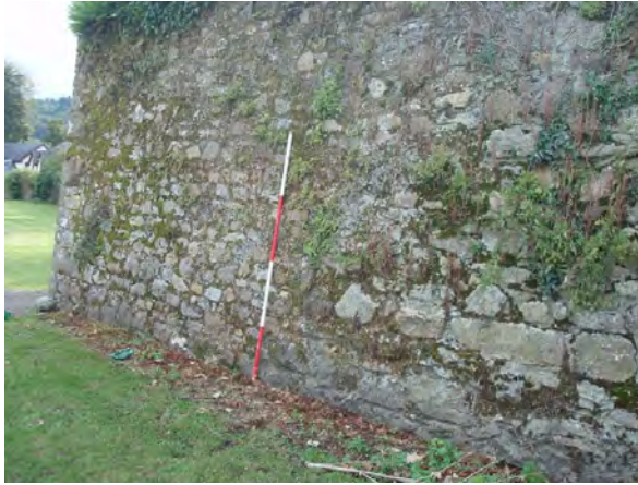
Plate 6. External view of town wall, showing original wall to right.
