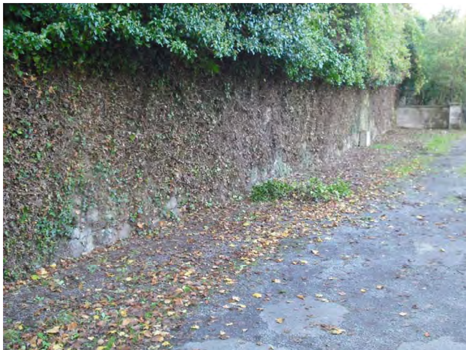
Picture 4 Elevation of Wall 'A' (with 2m of ivy removed)
