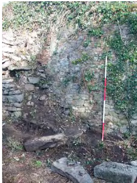
Plate 4. Wall walk with lowest step uncovered.
