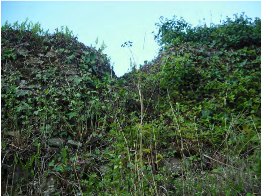
Picture 7 Opening in Wall A Parapet?
