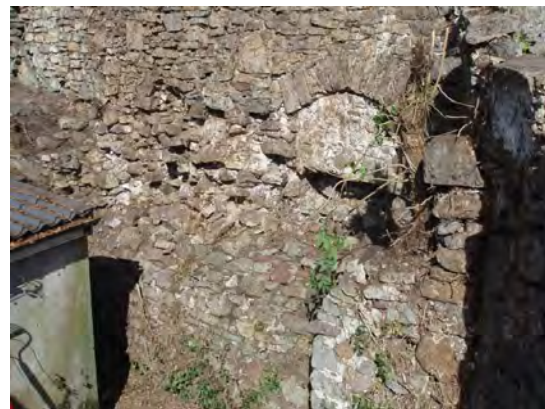
Plate 8. Blocked door ope.
