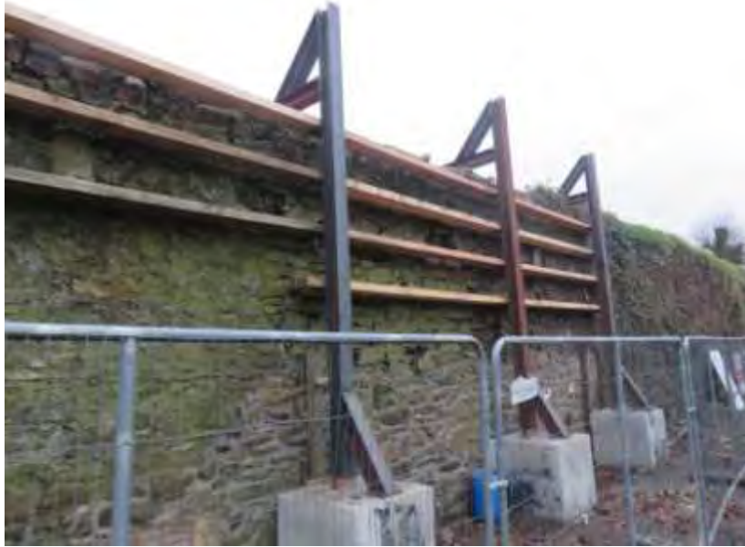
Fig. 17) The temporary shoring erected to the north elevation.
