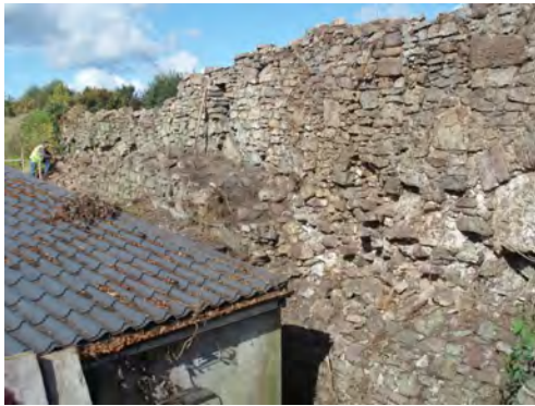
Plate 11. Wall walk inside, north wall.
