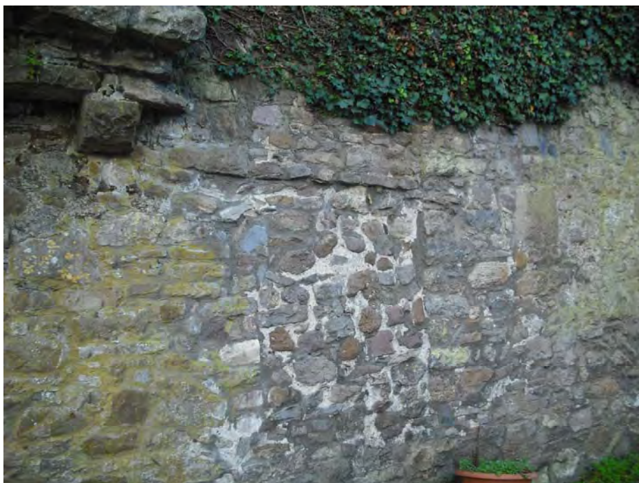
Picture 2 Old Opening Wall A
