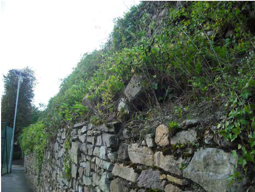
Picture 9 Tennis Court Side Loose Random Rubble on Ledge
