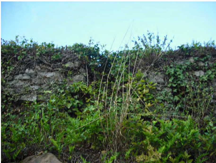
Picture 8 Opening in Wall A Parapet?
