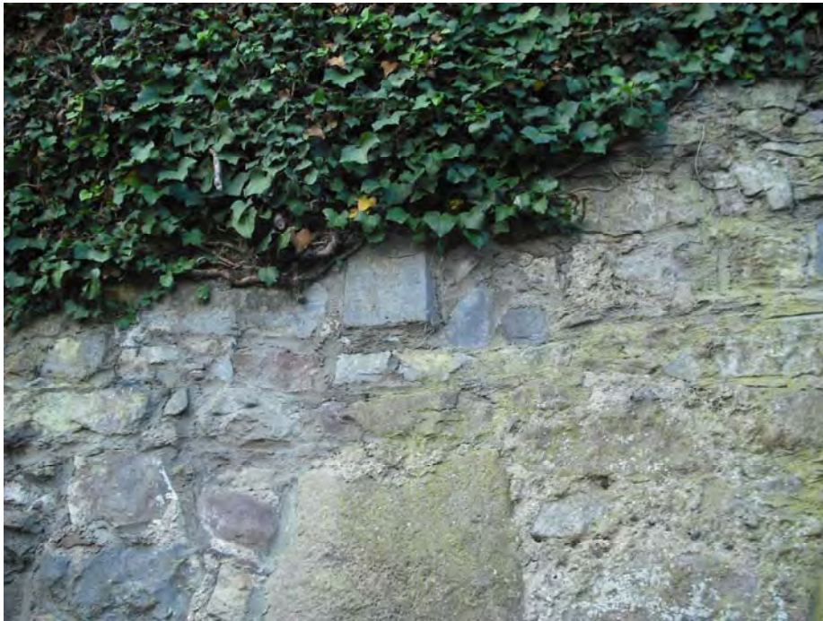
Picture 3 Piece of Ashlar/ Dressed Stone in Wall A
