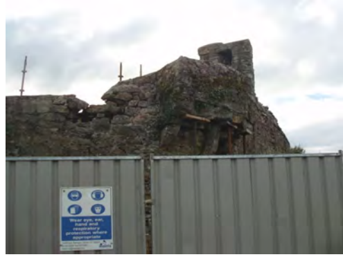
Plate 14. External view of propped bartizan.
