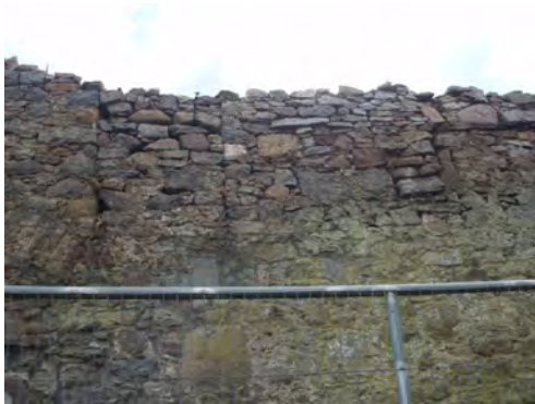
Plate 15. North wall, external, blocked opes.
