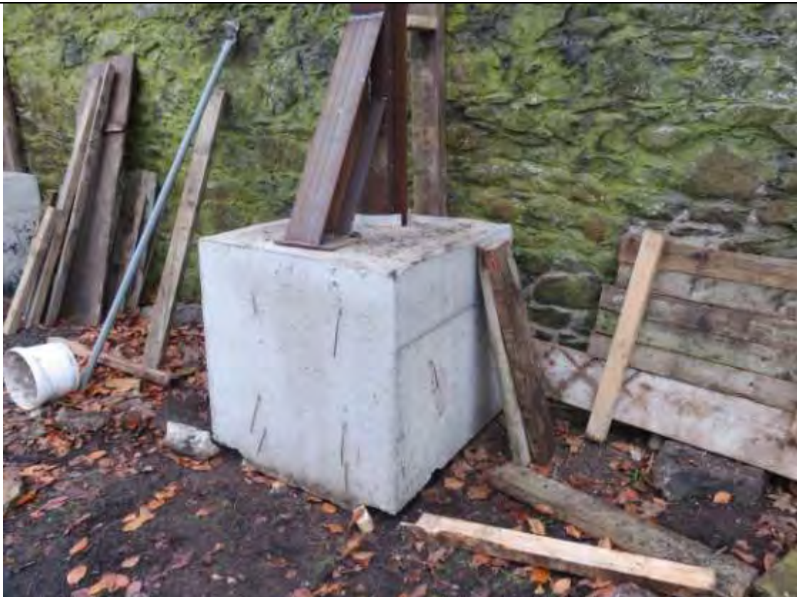
Fig. 20) The precast concrete base to support the metal work.
