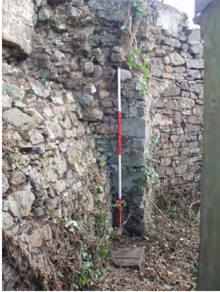
Plate 9. Projecting masonry, north wall.
