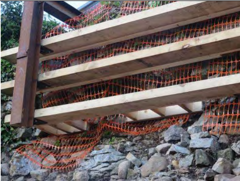
Fig. 23) The timber bracing was made to measure.
