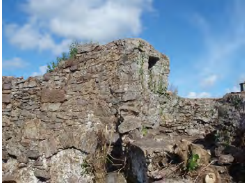
Plate 13. Bartizan, infilled opes of building.
