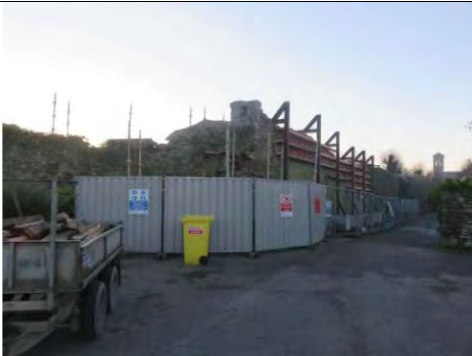
Fig. 21) A view of the north facing elevation.
