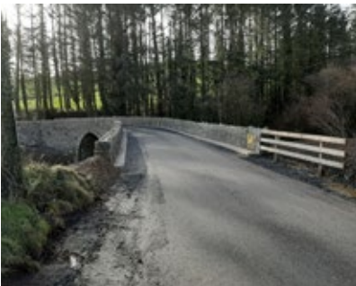
Killoskehan Bridge on the L-3216-20
