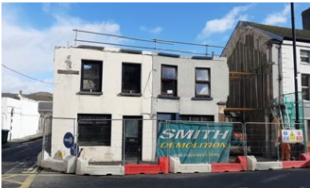
Emmet Place during demolition works
