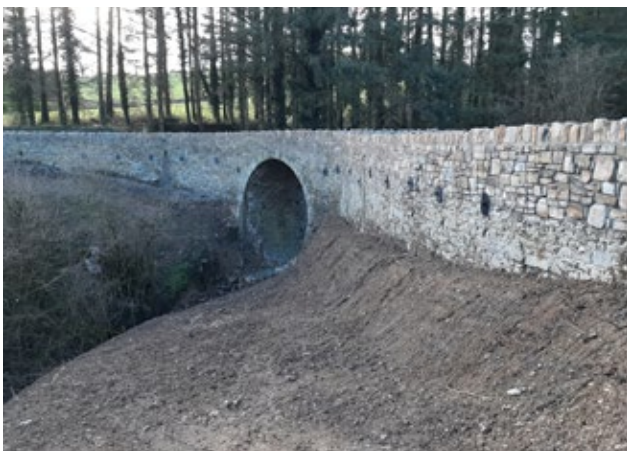
Bridge Rehabilitation works at Kiloskehan Bridge, Gortagarry
