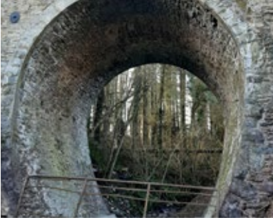
Killoskehan Bridge on the L-3216-20
