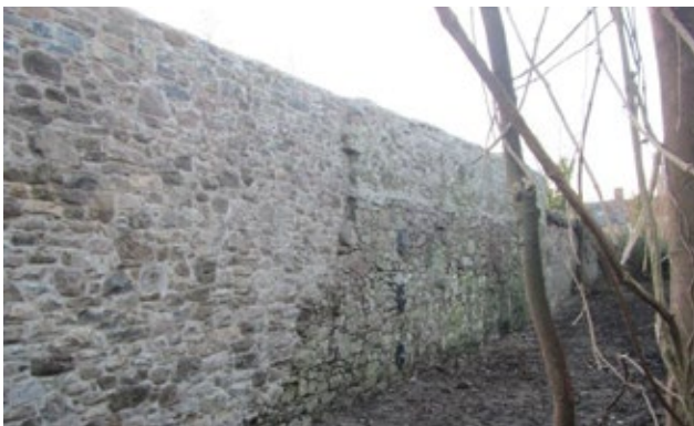
Works complete at Carrick on Suir
