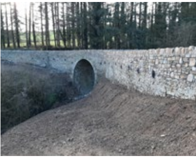
Killoskehan Bridge on the L-3216-20
