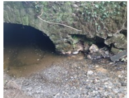
Curraghscarteen Culvert near Fethard
