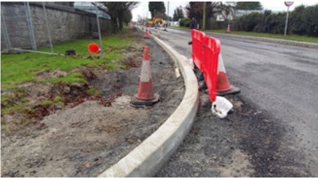
Works underway at Templemore November 2020
