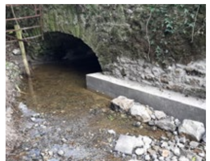
Curraghscarteen Culvert near Fethard
