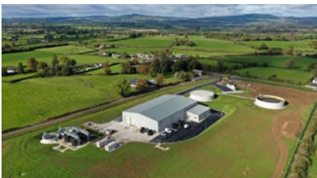
Thurles RWSS - Water Treatment Plant
