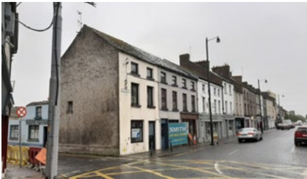
Emmet Place before demolition works
