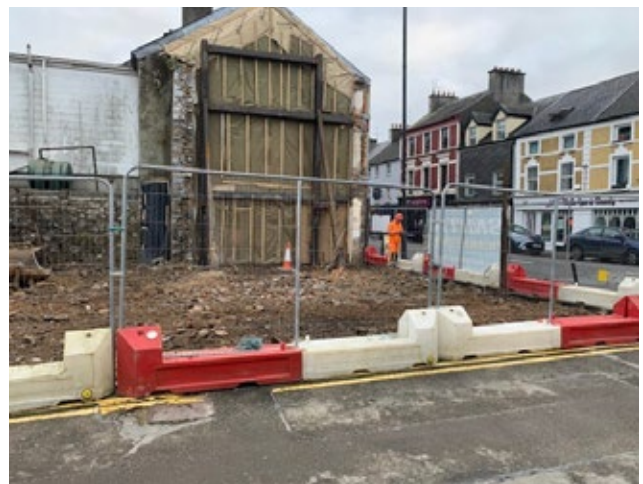
Emmet Place after demolition works
