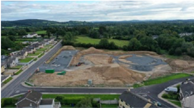
Aerial view of works at Newport Town Park
