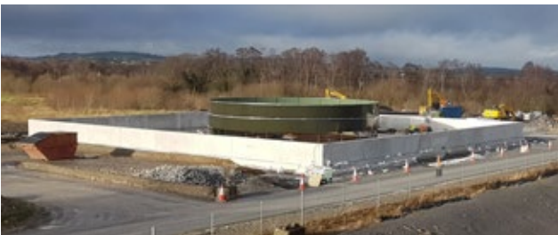
2020 leachate holding tank under construction
