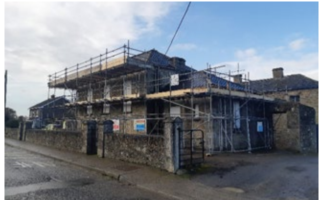
Newport Courthouse - works substantially completed
