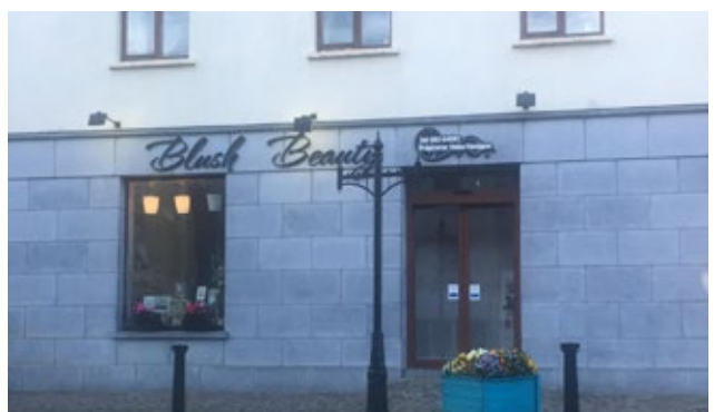
Ladyswell Street, Cashel - Photos before and after works
