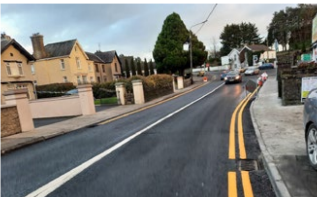
Pavement Works at Birr Road Roscrea
