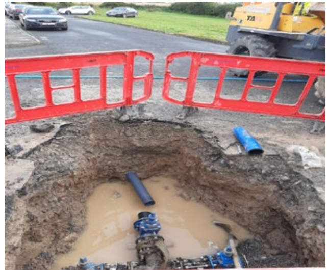
Templetuohy Watermain Rehabilitation
