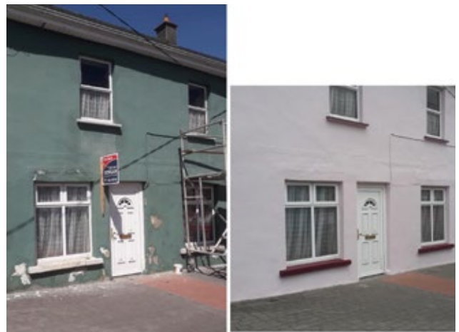
Photos before & after works
