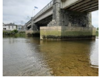
Dillon Bridge, Carrick on Suir
