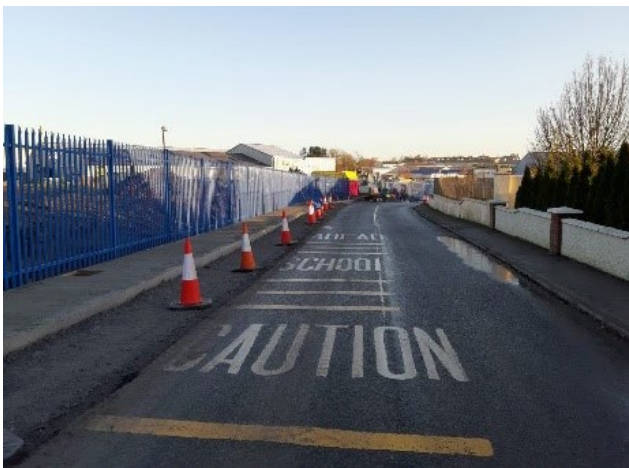
Safety Improvement Works at Windmill Road, Cashel
