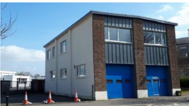
Training Centre Thurles which was made operational in March 2020
