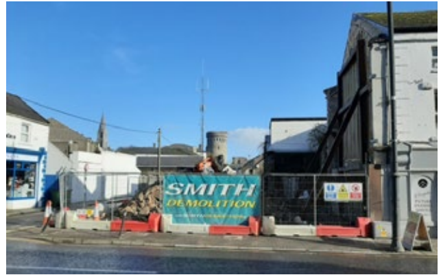
Emmet Place after demolition works
