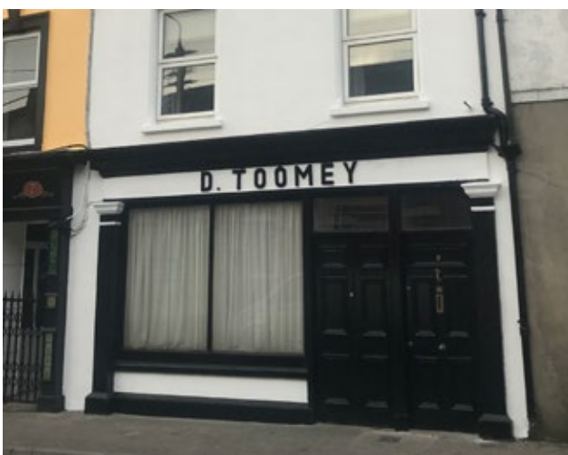
No. 8 Davis Street, Tipperary - Photos before and after works
