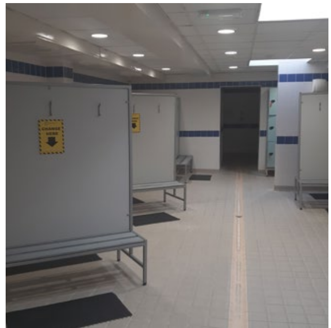
Photo of Refurbished Pool Changing Room
