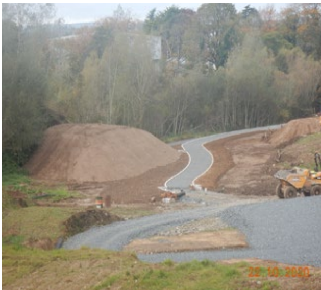
Works to Riverside Path at Bandstand Junction in Newport Town Park
