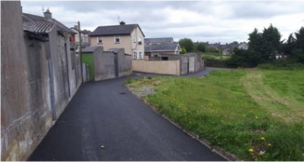
Reinstatement of Chaple Lane, Roscrea (GMA Funded Works)
