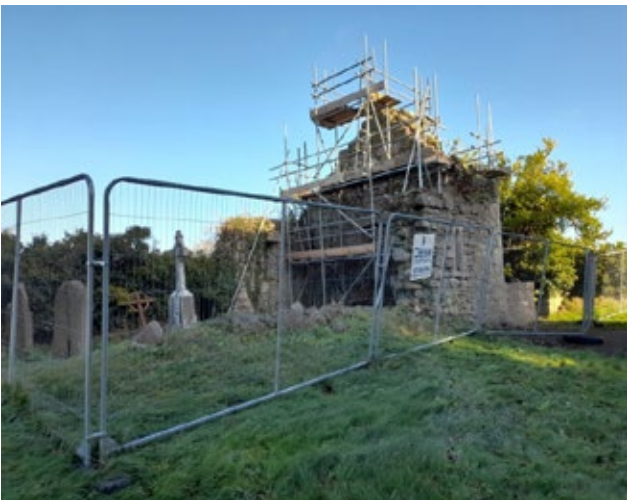
Works in progress at Pallas Church
