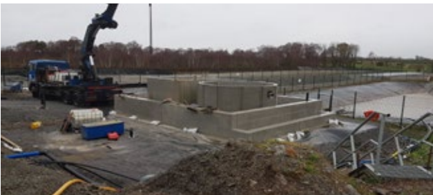
2020 leachate pumping station under construction
